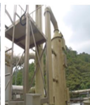
洗滌塔(鹼排) Scrubber (Emissions of alkali air)
