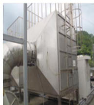
吸附塔 Adsorption tower
