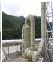
洗滌塔(酸排) Scrubber (Emissions of acid air)
